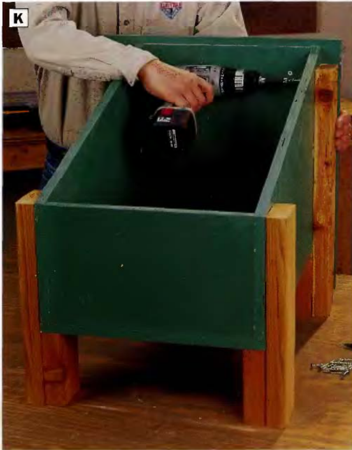
PHOTO K: Install the leg assemblies to the cart box with 1½-in. screws. The front legs should butt against the back of the cart face. Attach the rear legs so they are flush with the cart back.
