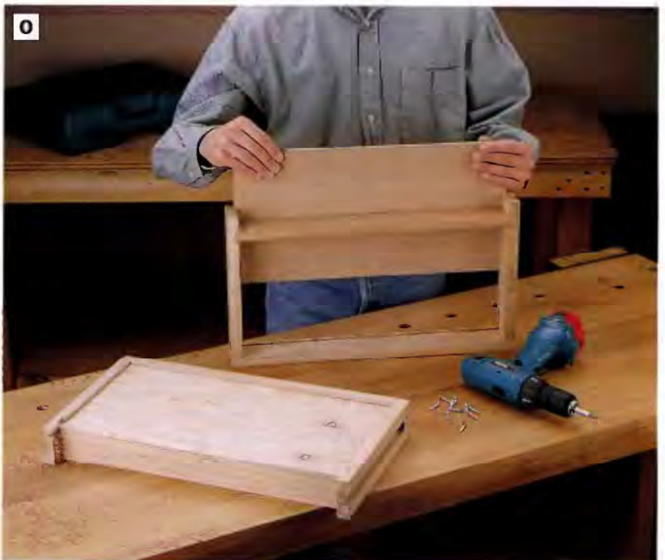
PHOTO O: Slide the drawer bottoms into the grooves in the drawer sides and front. Secure the drawer bottoms with three screws driven through the drawer bottom and into the bottom edge of the drawer back. Do not use glue.
