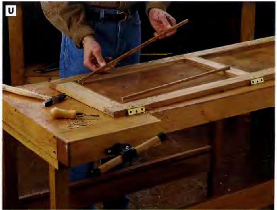
PHOTO U: Set the glass panels in place in the doors and secure them with ¼ × ¾-in. oak retainer strips. Use 1-in. wire brads driven into pilot holes to fasten the strips to the inside edges of the rabbet grooves in the door frames.
