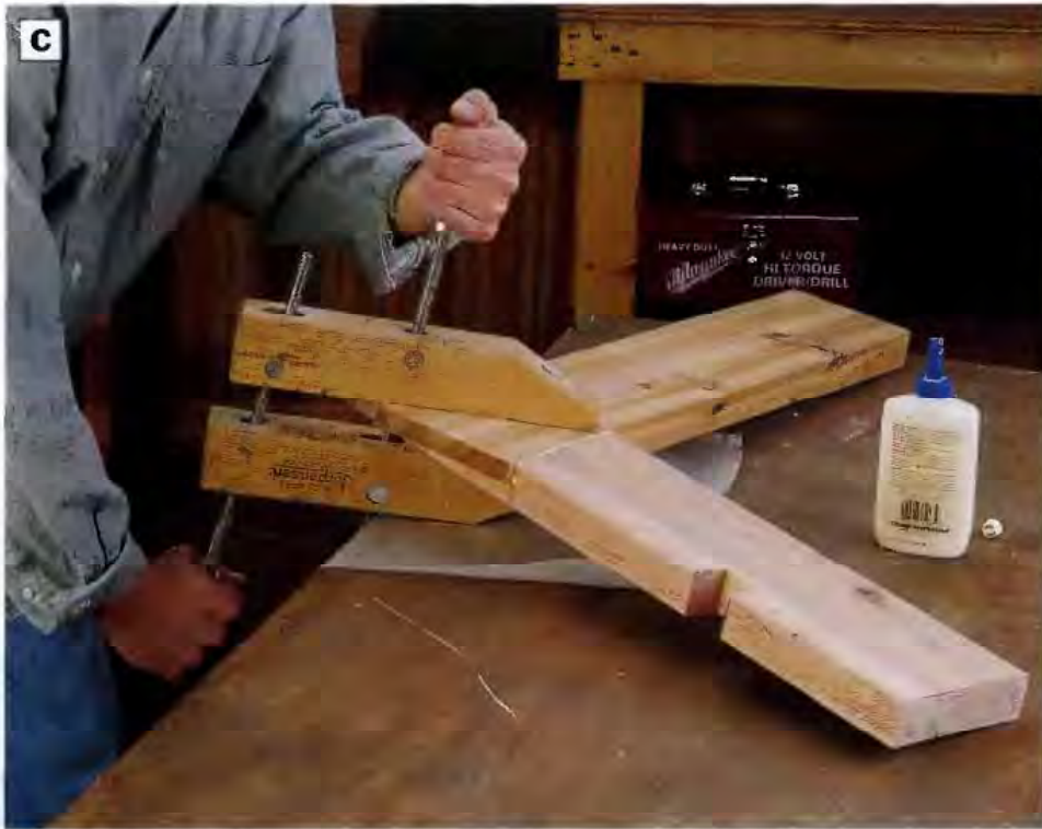
PHOTO C: Glue and clamp the half-laps of the seat supports and the back supports together to create L-shaped blanks for the three support structures. Use weatherproof glue.
