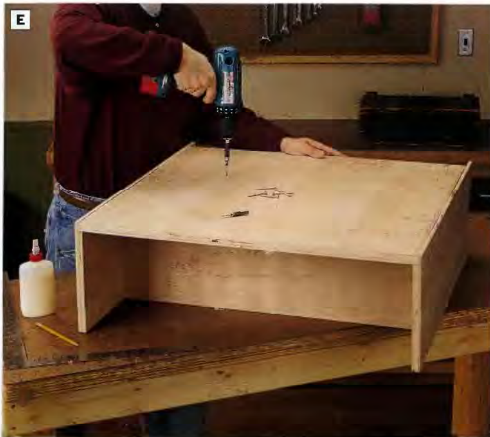
PHOTO E: Install the back on the bookcase with glue and screws driven into the back edges of the shelves. Mark the shelf locations on the back first, so you can drive the screws accurately.
