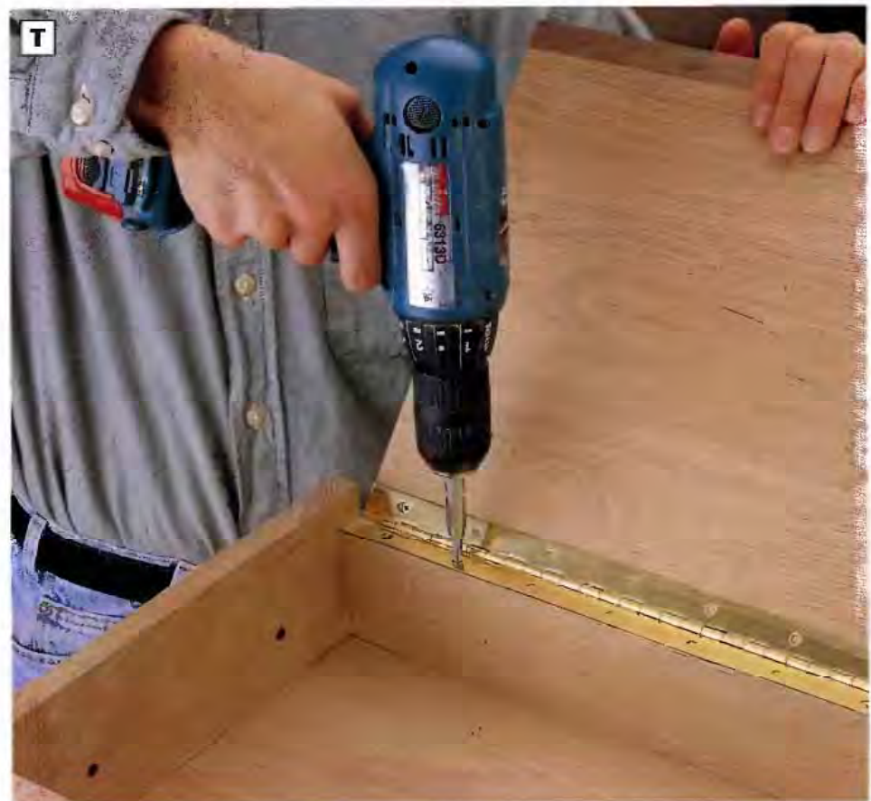
PHOTO T: Dry-fit the lid by attaching the piano hinge with one or two screws in each end and another in the middle. Remove the hinge, once you're satisfied that everything fits together, and reattach it after the finish is applied.
