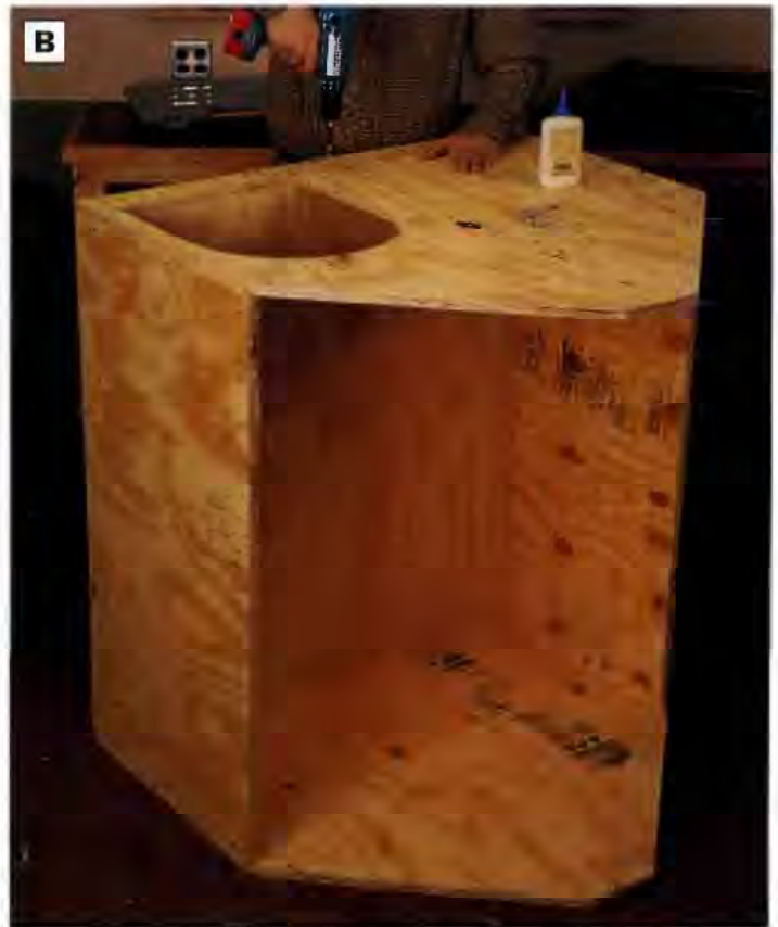
PHOTO B: Fasten the bottom panel in place between the front, back and side pieces with countersunk deck screws. Position the bottom 3 in. up from the bottom edges of the parts and so the top face is flush with the bottom of the door opening.
