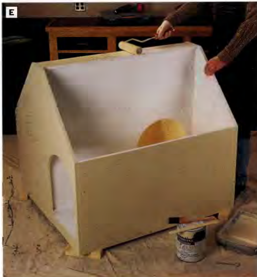
PHOTO E: Prime and paint the doghouse surfaces, inside and out. Seal the bottom edges with primer and paint, to keep the plywood from wicking up ground moisture.
