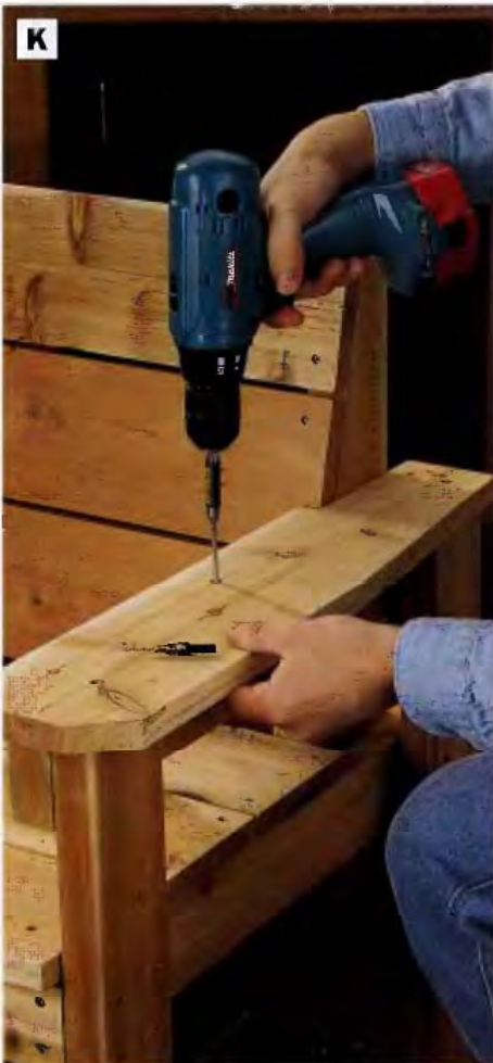
PHOTO K: Position the arms on the leg assemblies and fasten them to the arm supports and the legs with screws.
