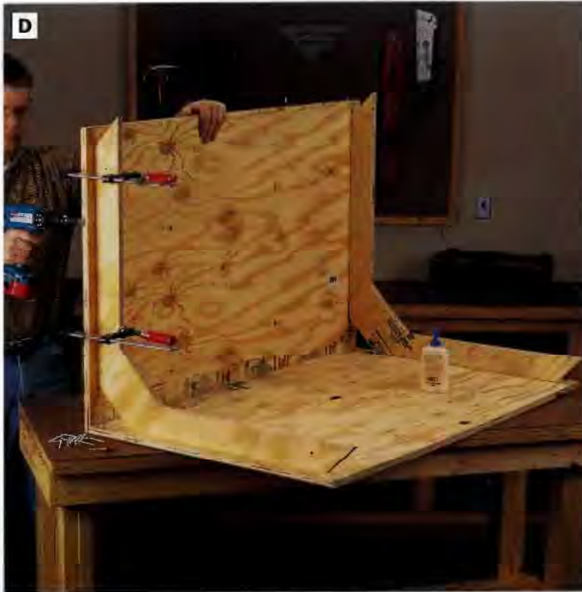
PHOTO D: Assemble the roof panels and gussets to form the roof structure. Allow for a 1-in. overhang between the ends of the roof and the gussets. Fasten the parts with glue and countersunk deck screws.
