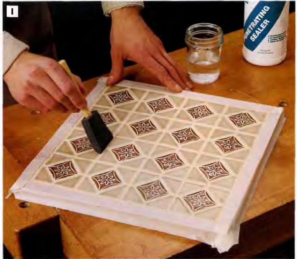
PHOTO I: Seal unglazed tile and grout joints with penetrating sealer. Use a disposable foam brush to apply the sealer. Because a plant stand is likely to be exposed to a considerable amount of moisture, sealer is important to protect the plant stand top and to help inhibit mildew and other forms of discoloration that can affect the grout.
