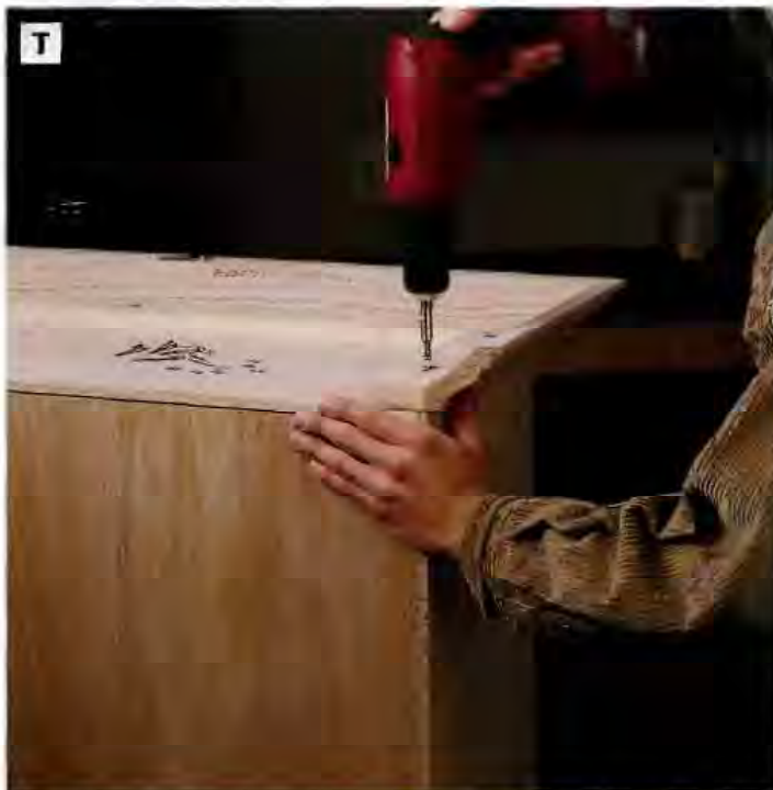
PHOTO T: Attach the crown frame to the top of the cabinet with screws and washers. The screw slots in the tops of the scrap wood backer frame allow for cross-grain expansion and contraction of the solid wood top.
