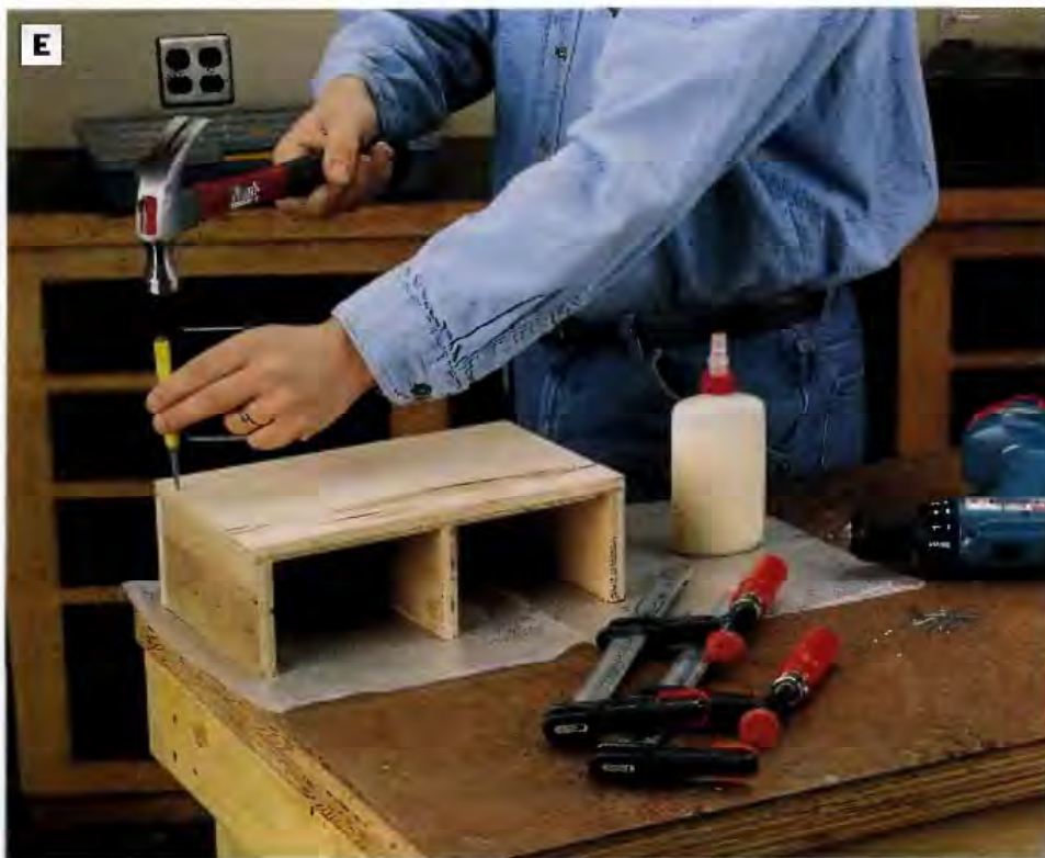
PHOTO E: Fasten the drawer sides and divider to the bottom and back with the drawer arranged upside down on your bench. Glue, clamp and nail these joints.
