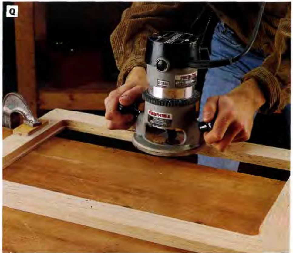
PHOTO Q: Rout a \frac{1}{4} \times \frac{3}{8} -in.-deep rabbet recess around the perimeter of each opening in the upper cabinet doors. Use a \frac{1}{4} -in. piloted rabbet bit (See page 137) to make the cuts. Square off the rounded corners left by the router bit, using a sharp chisel. To keep the wood from tearing, score along the chisel lines with a sharp knife before squaring the corners.
