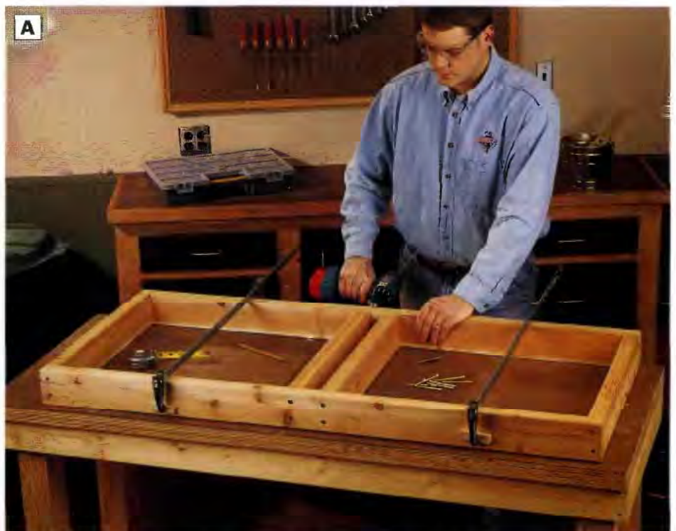
PHOTO A: Build the bench seat frame by fastening the front, back, ends and two stretchers together with 3-in. countersunk deck screws.
