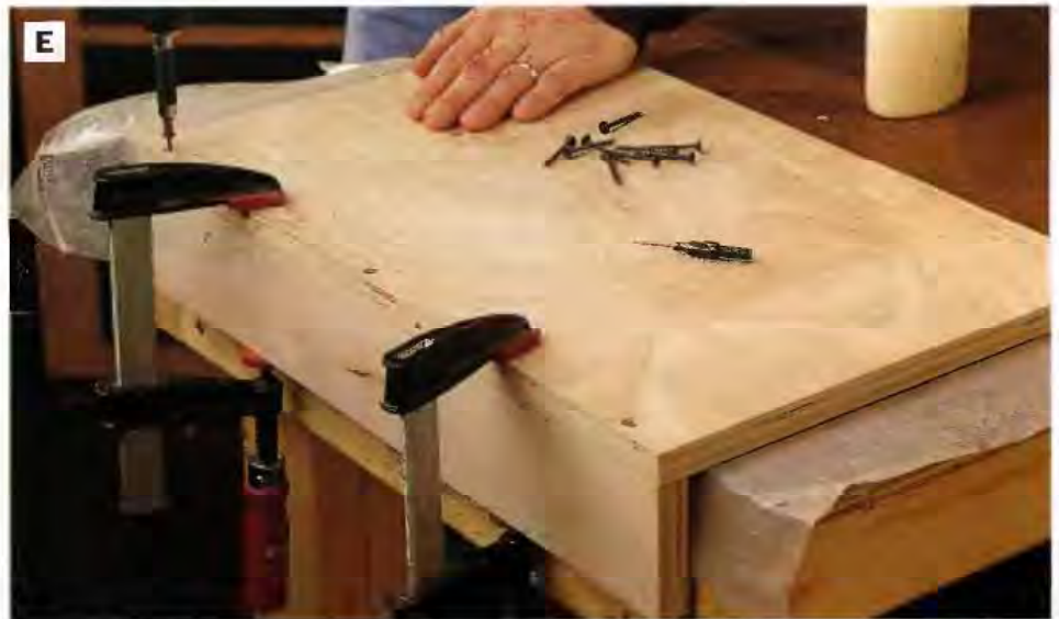
PHOTO E: Spread glue along one edge of the shelf back and clamp it flush with the back edge of the shelf. Attach the parts with countersunk 2-in. drywall screws.
