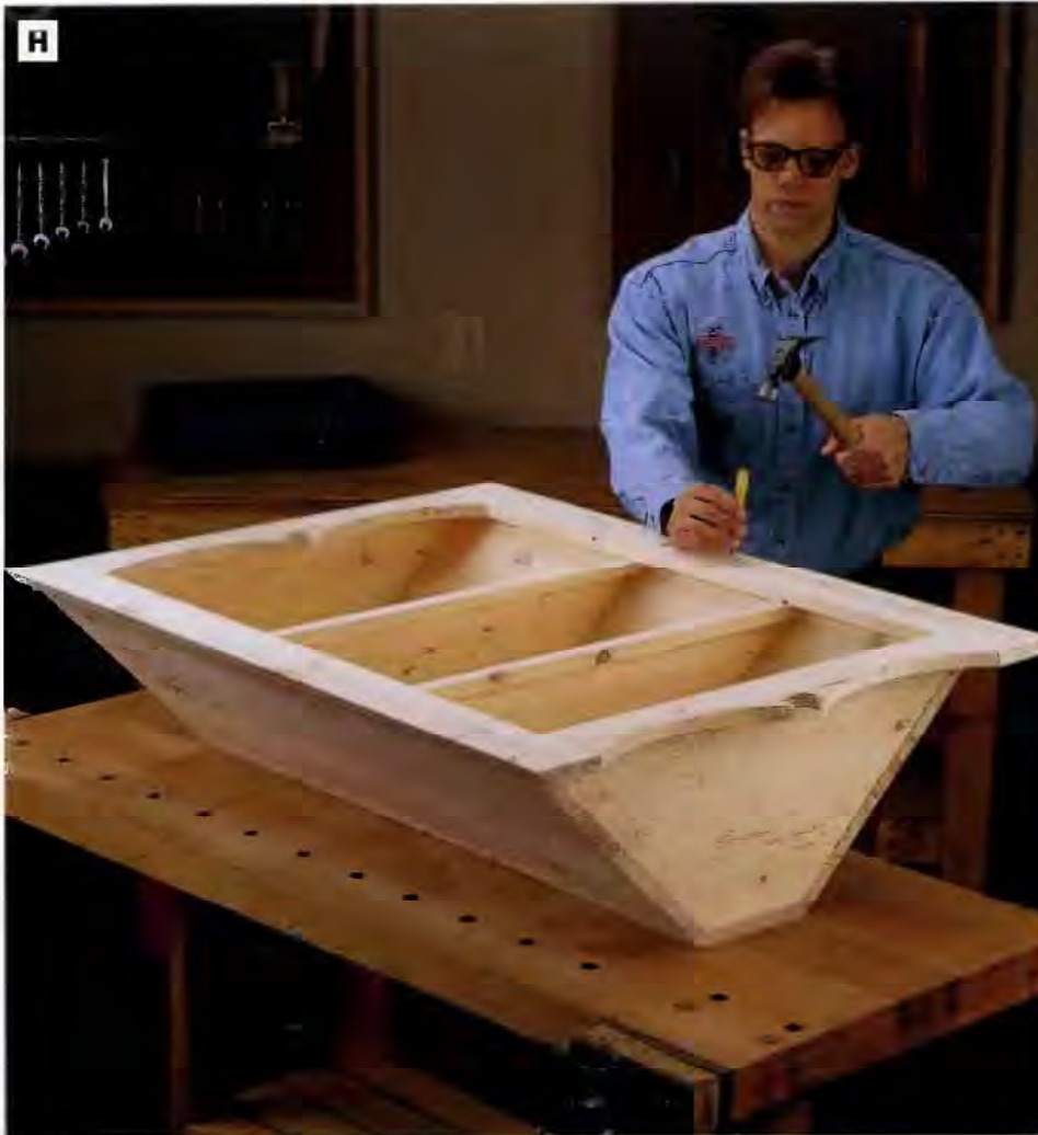
PHOTO H: Attach the face frame to the cupboard carcass with glue and 4d finish nails. Drive the nailheads below the face frame surface with a nailset.
