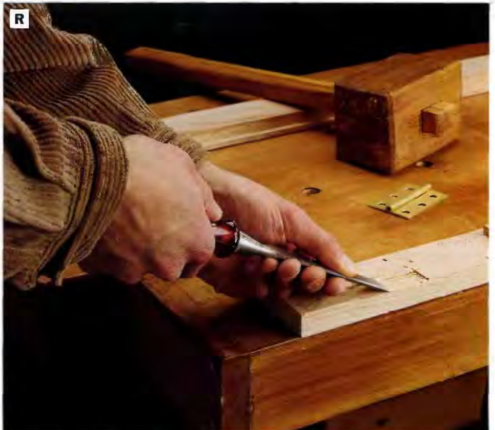
PHOTO R: Chisel mortises for the hinges into the inside faces of the outer door stiles and into the front edges of the cabinet sides. Use one of the leaves from the 2\frac{1}{2} -in. butt hinges as a template for tracing the cutting lines for the mortises.
