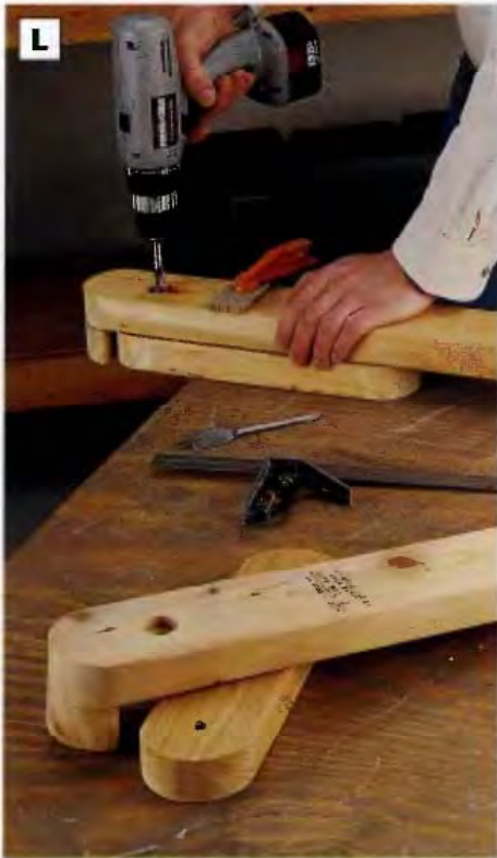
PHOTO L: Drill holes through the foot rest rails and the legs. The parts will attach with bolts so the legs can pivot on the rails.
