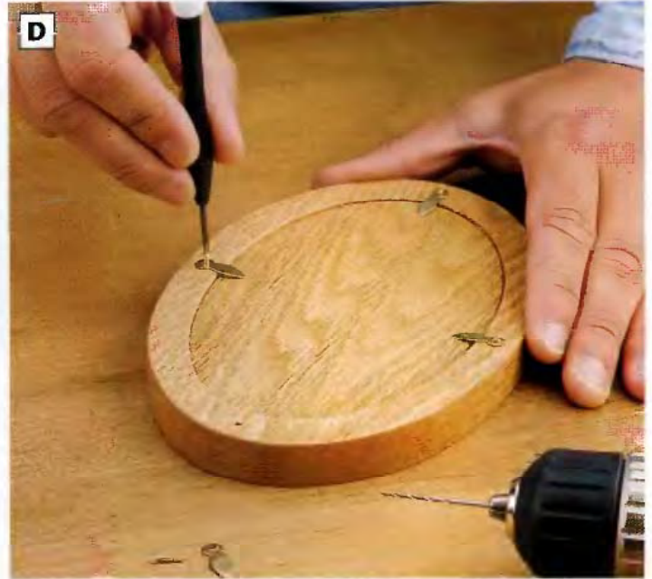
PHOTO D: Four brass turn buttons hold the glass, photo and back in the frame. Install the hardware so the turn buttons are spaced evenly around the frame. Drill pilot holes for the tiny turn button screws.
