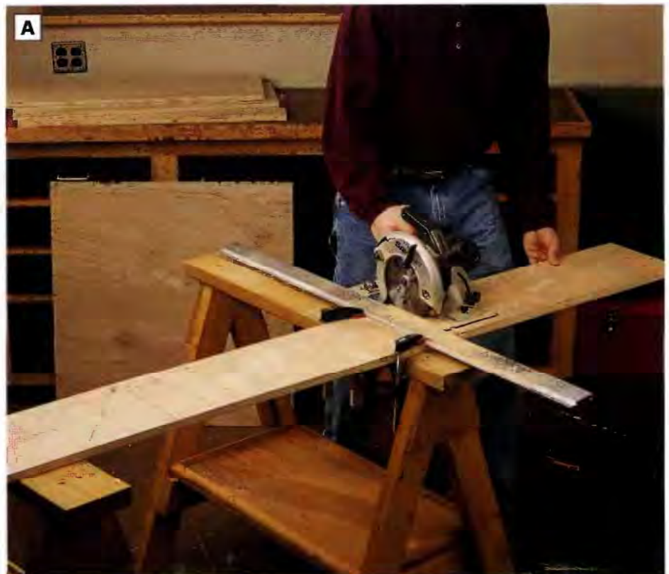
PHOTO A: Lay out the bookcase parts on the plywood sheet, then rip and crosscut them to size. We arranged the shelves end-to-end on the plywood so we could rip one long strip, then crosscut the strip twice to form the three shelves.
